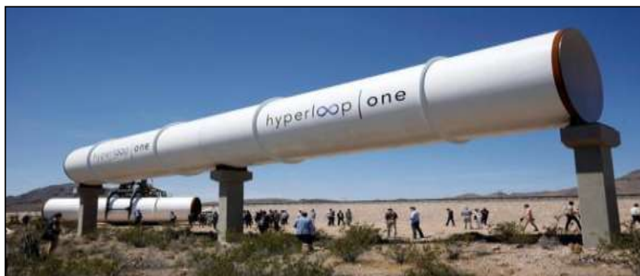
Fig. 27 : Hyperloop test track under construction – Picture: Reuters
