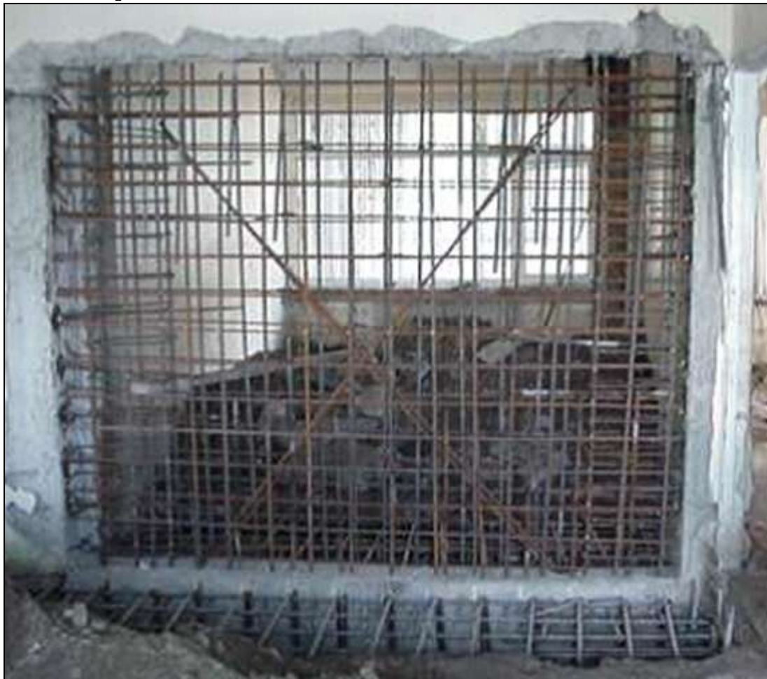
Fig 47: Additional Shear Wall
